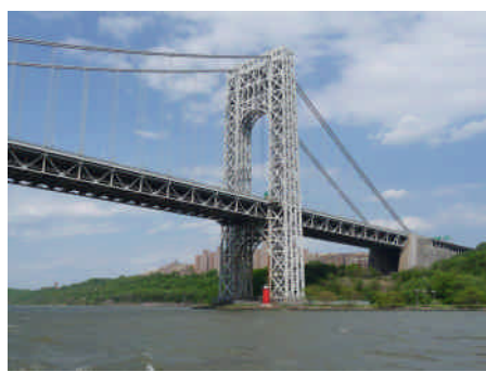
George Washington Bridge
